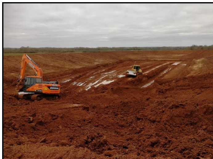
Digging the reservoir
