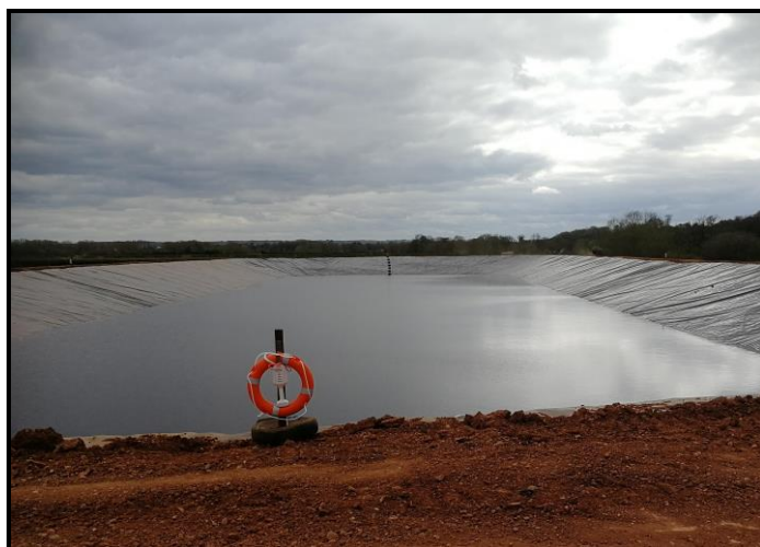
Reservoir after lining
